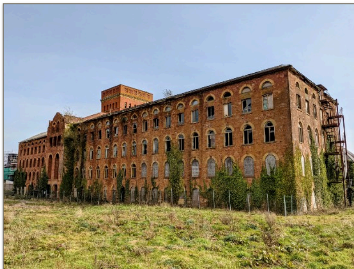
Historic... The old section of Tonedale Mill
