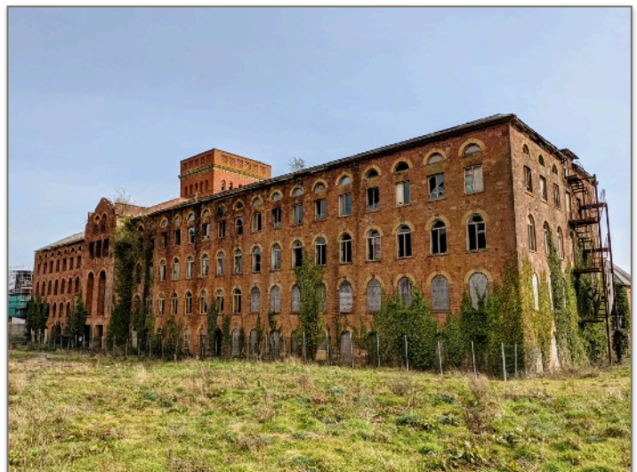
Historic... The old section of Tonedale Mill
